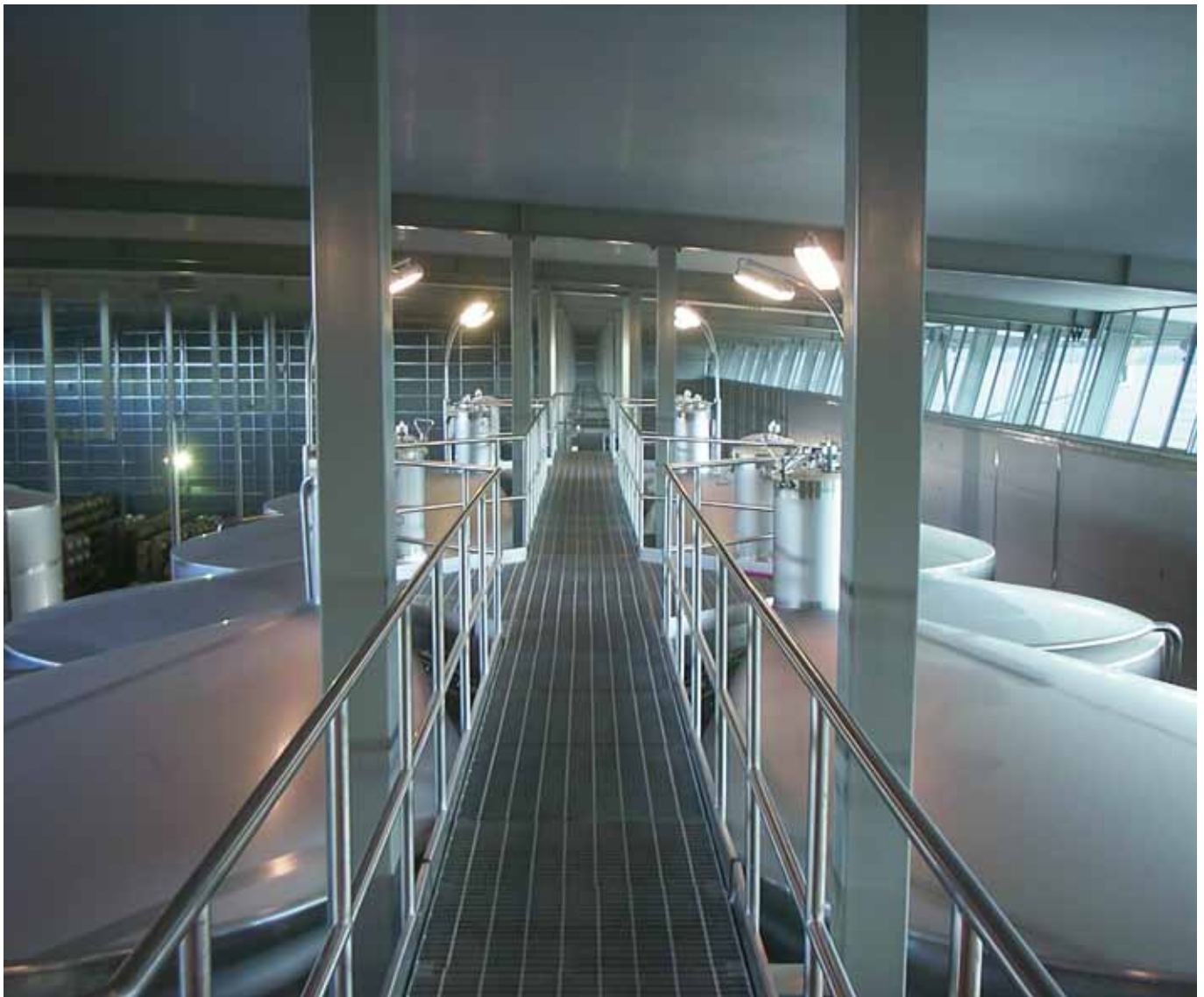
Diamond walkways across storage tanks
