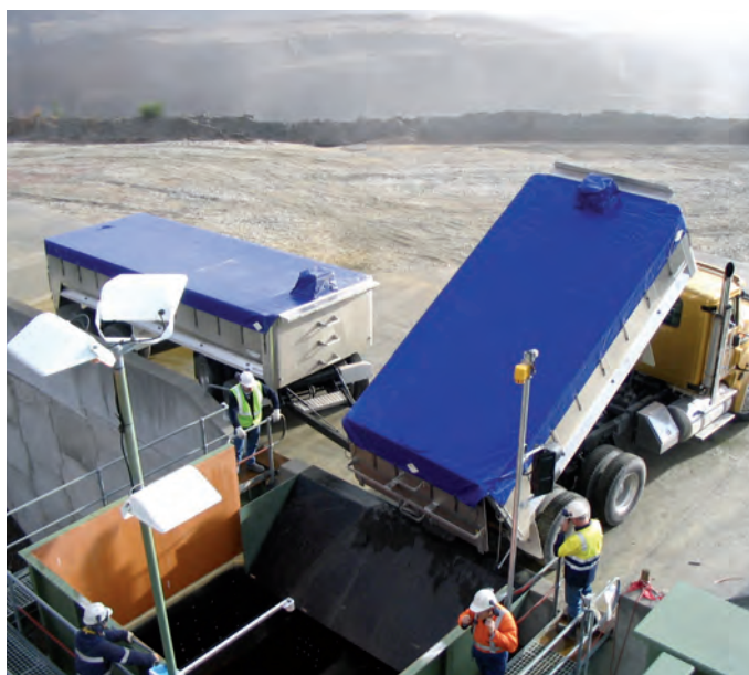
Concentrate receival hopper being loaded
