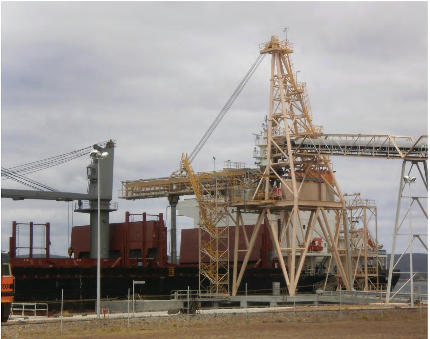
Brightwater designed an all-weather truck reception system for receiving of pellets, a shuttle conveying system to distribute pellets within the building, and a reclaiming system to connect the storage building with the existing ship loading infrastructure.
