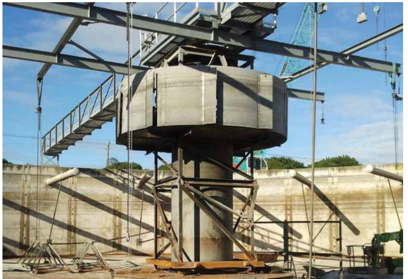
One of the four clarifiers being repaired
