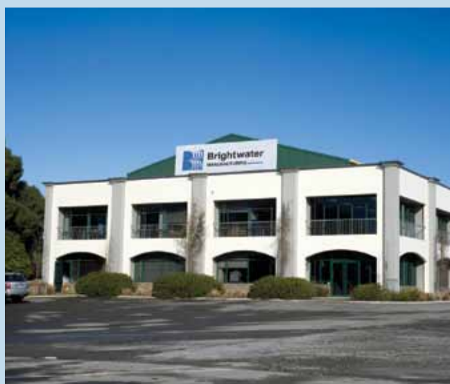
Brightwater's Christchurch facility
