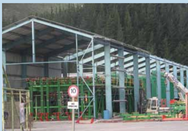
Kaituna Mill Bin Sorter during installation
