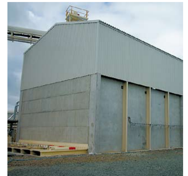
CHH LVL 1000m 3 Push Floor Bunker
