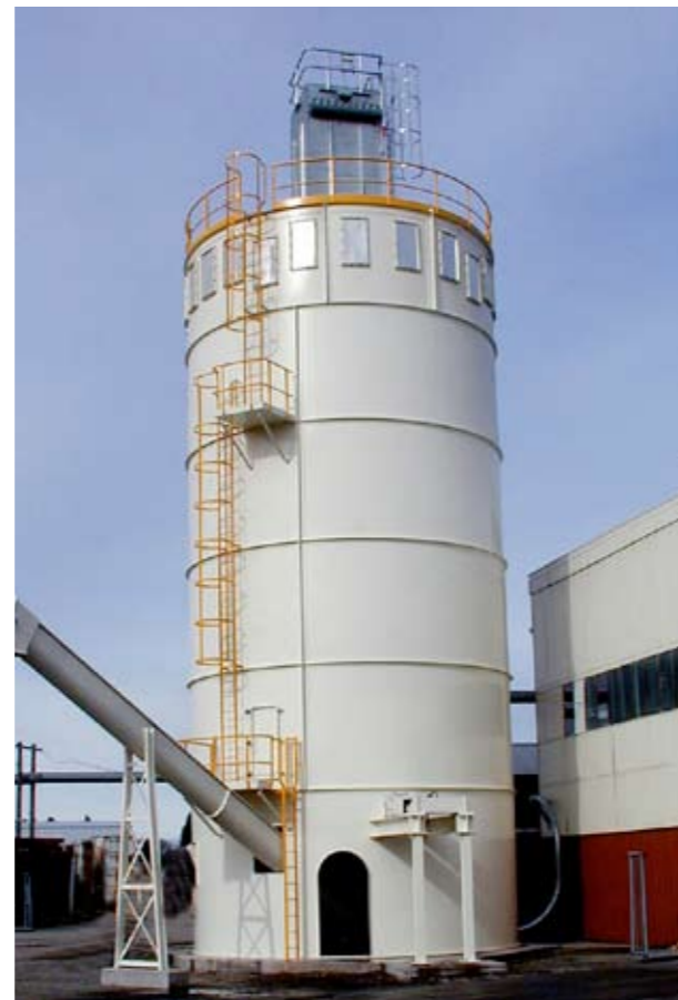
KLC 400m 3 Silo with truck loading screw
