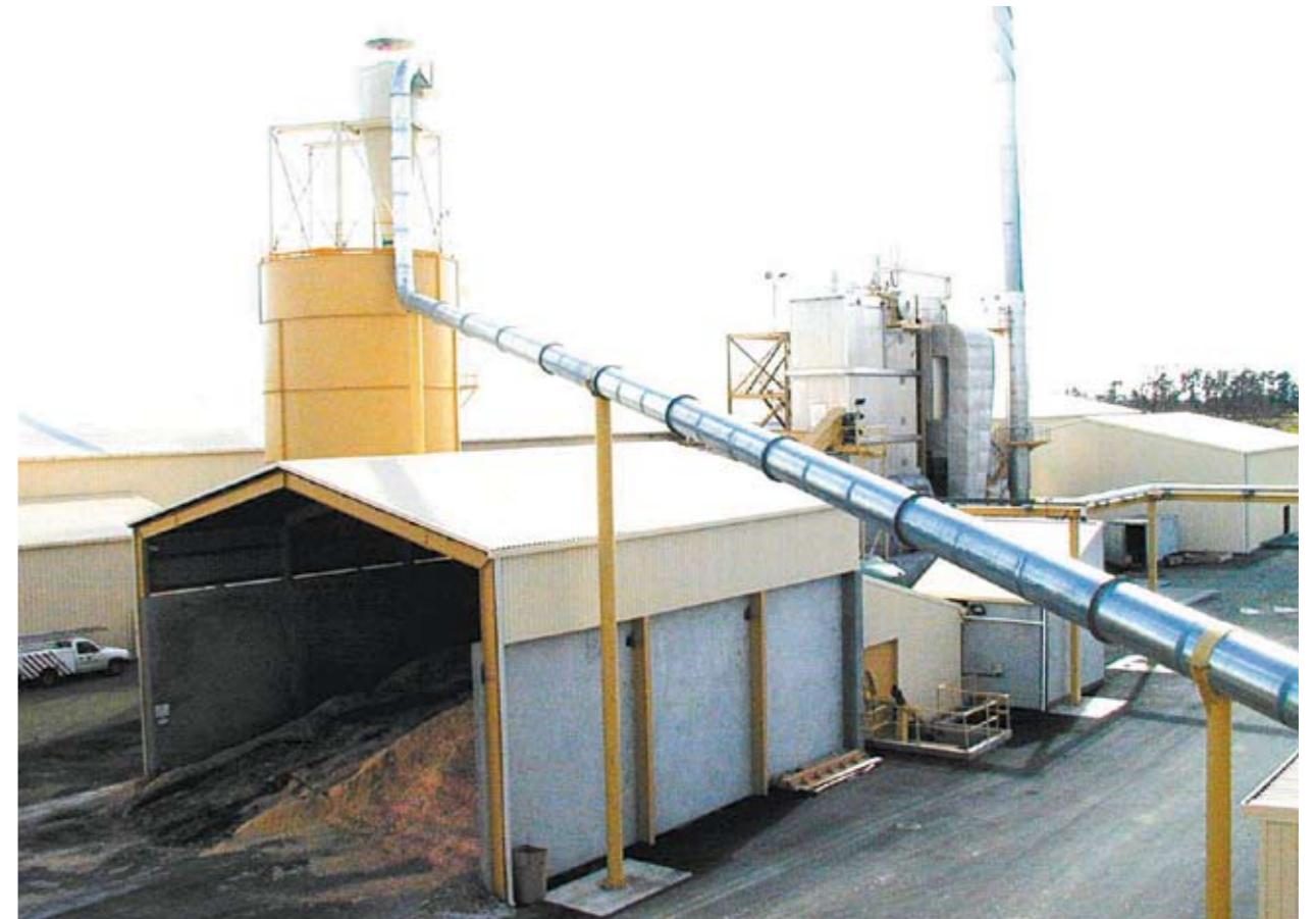
JNL Kaitaia 800m 3 Pull Floor Bunker
