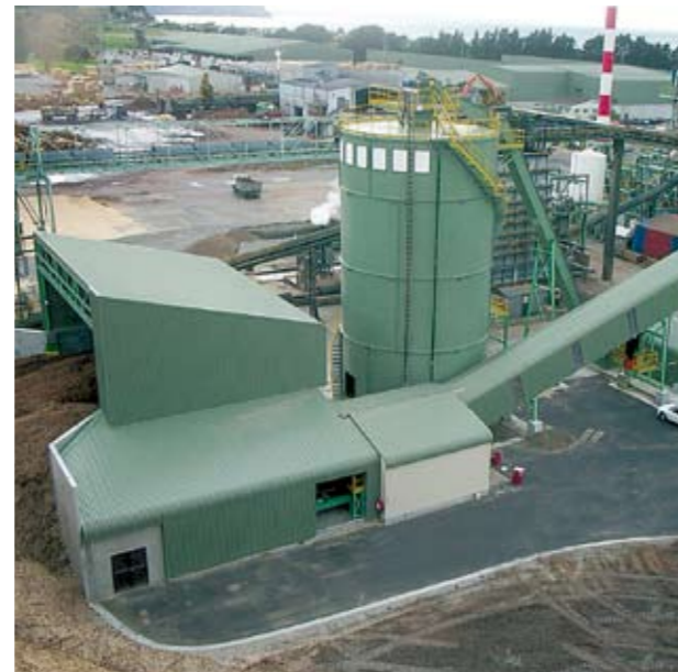
800m 3 Circular Screw Reclaimer Silo
