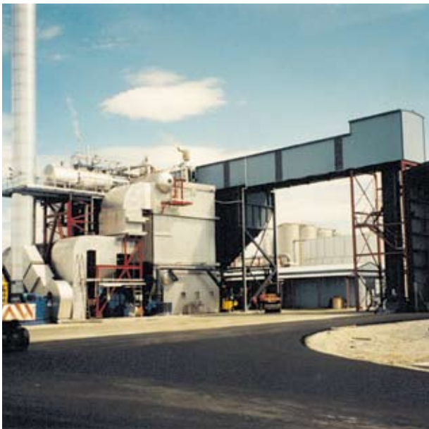
Alpine Dairy Coal Reception and conveying System incorporating a 160m 3 Pull Floor Reception Bunker
