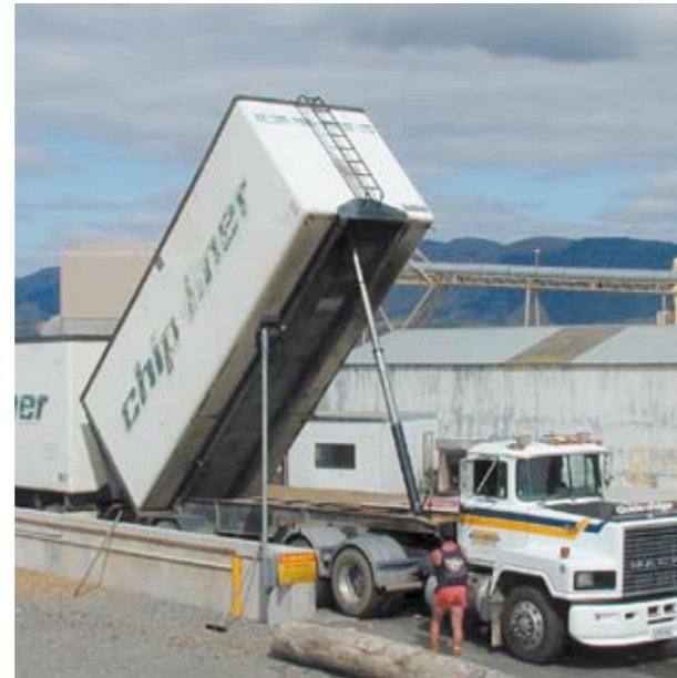
NPIL Chip Reception Bunker - 150m 3 Double Push Floor
