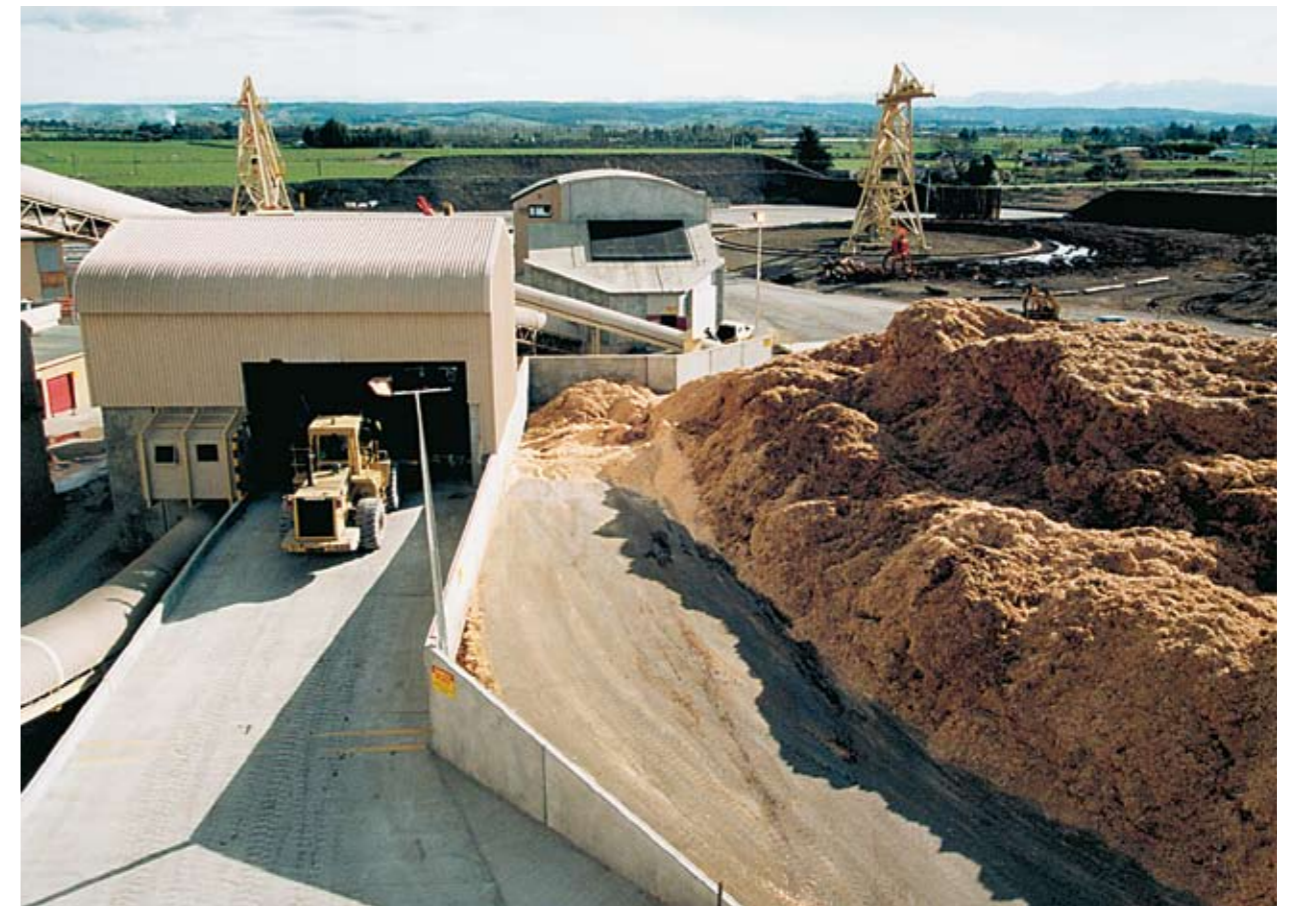
NPIL 800m 3 Silo
