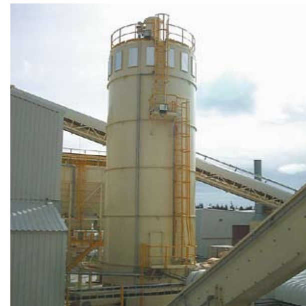
CHH LVL 200m 3 Silo
