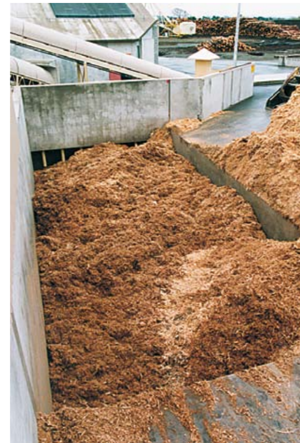
NPIL Imported Fuel Reception 250m 3 Push Floor Bunker
