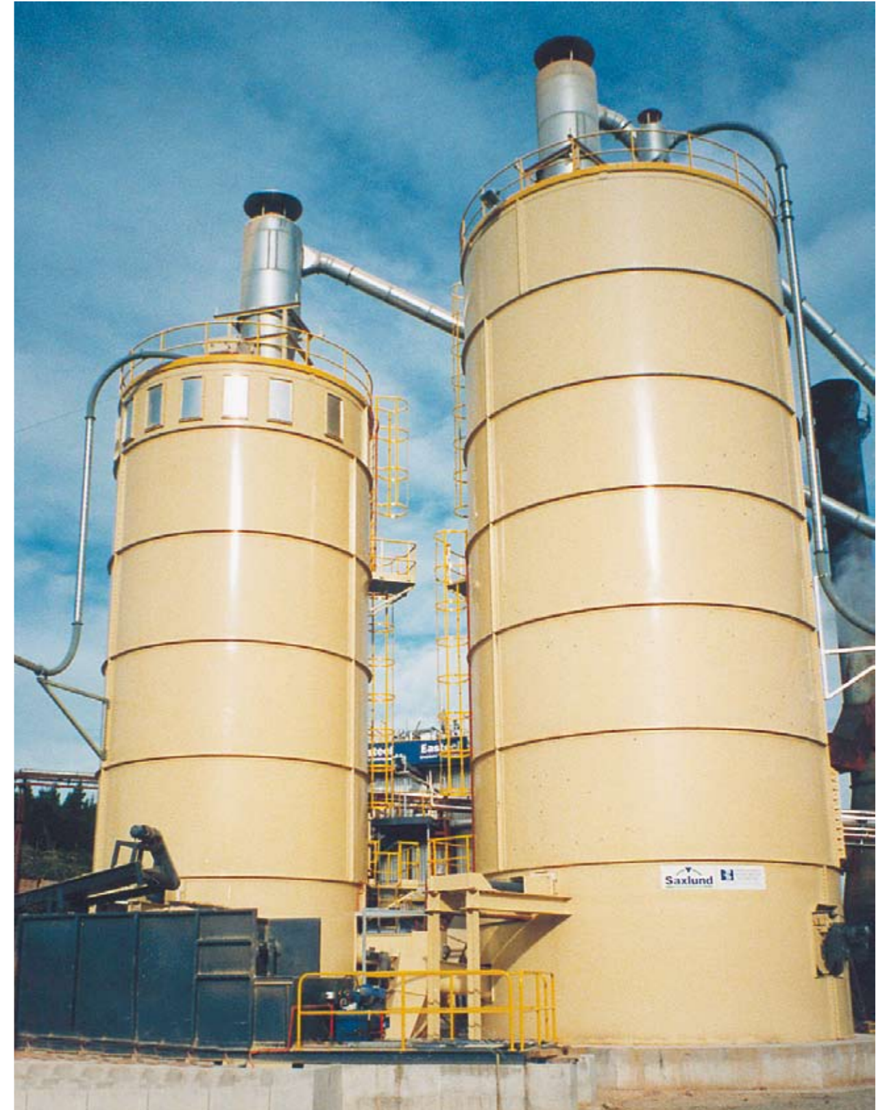
BML 275m 3 and 550m 3 Silos and 20m 3 Pull Floor Bunker
