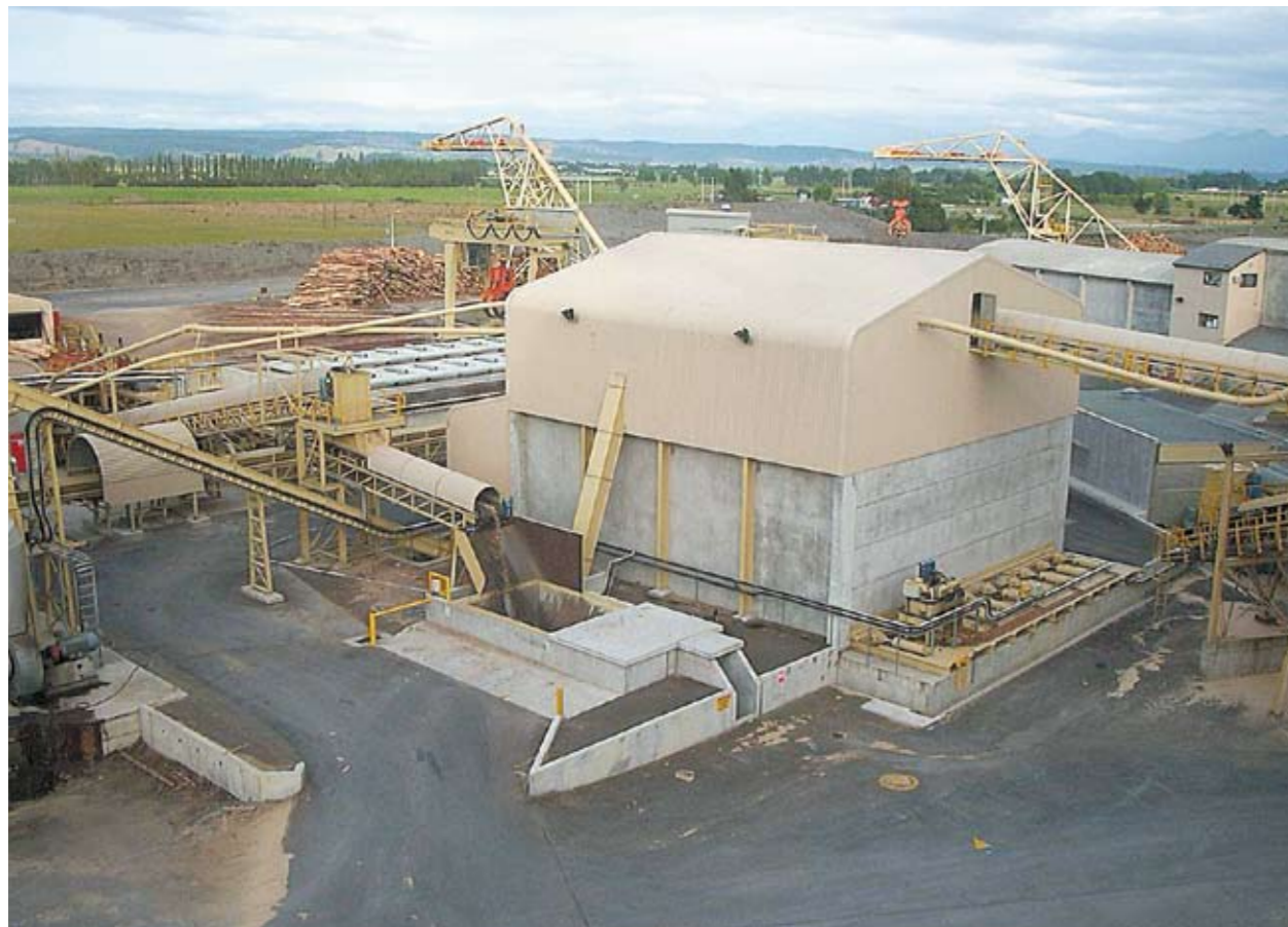
NPIL 1500m 3 Push Floor and En Masse Conveyor
