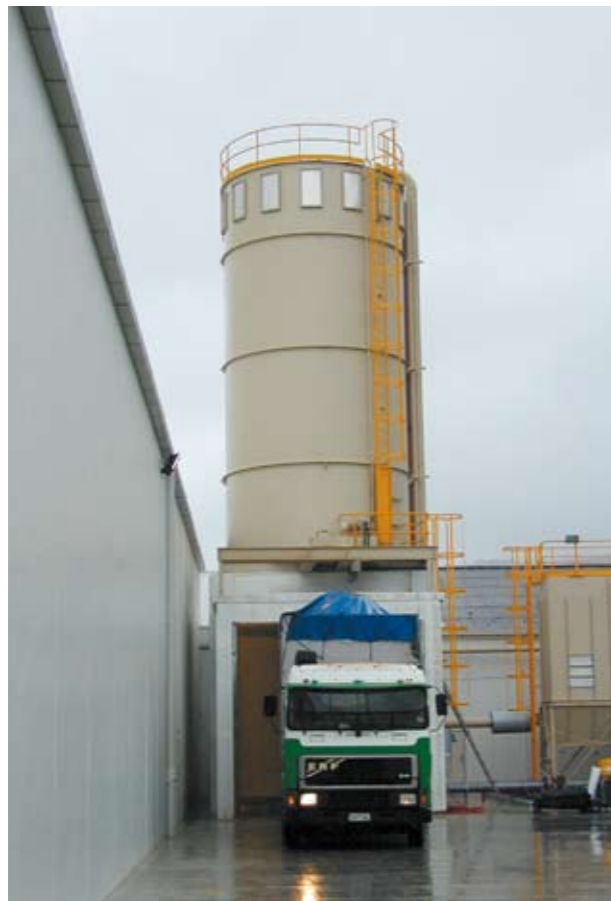
Claymark Industries' 200m 3 portal mounted silo
