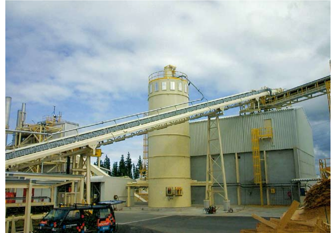
Carter Holt Harvey LVL plant, Marsden Point
