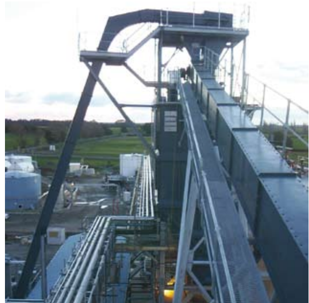
Clandeboye Coal Handling, Fonterra
