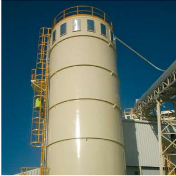
McAlpines 250m 3 Silo
