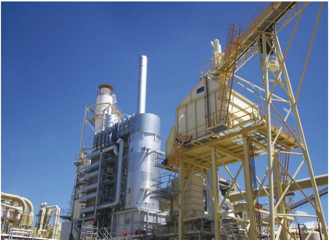
Elevated Fuel Metering System
