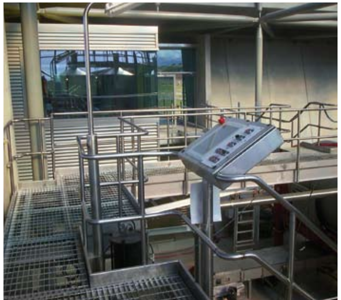
Looking from upper de-stemmer platform to receival office
