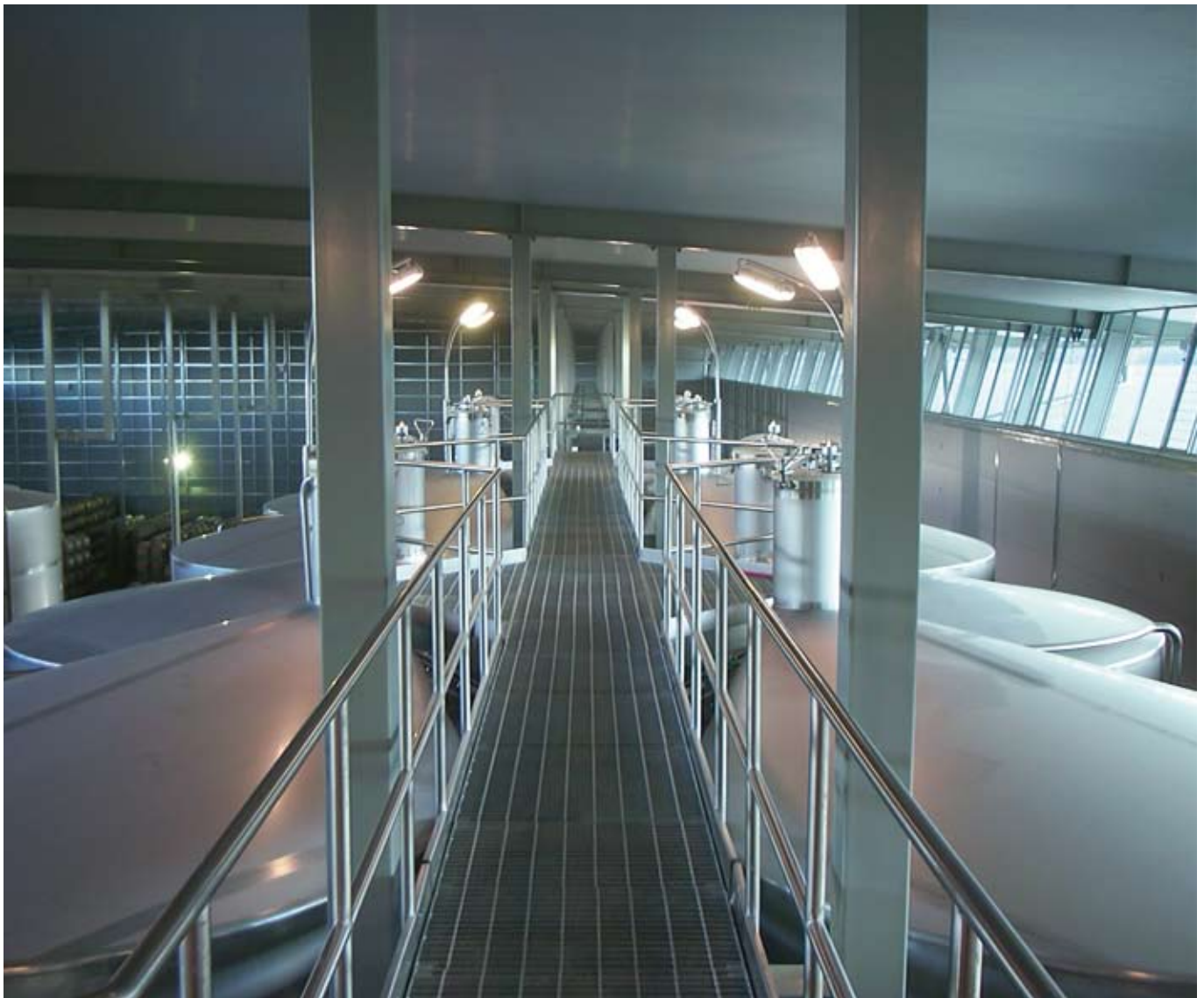
Diamond walkways across storage tanks
