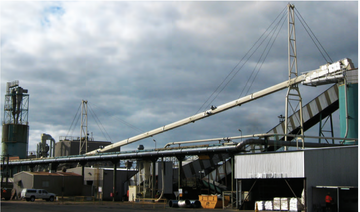
Completed Installation (Side View)
