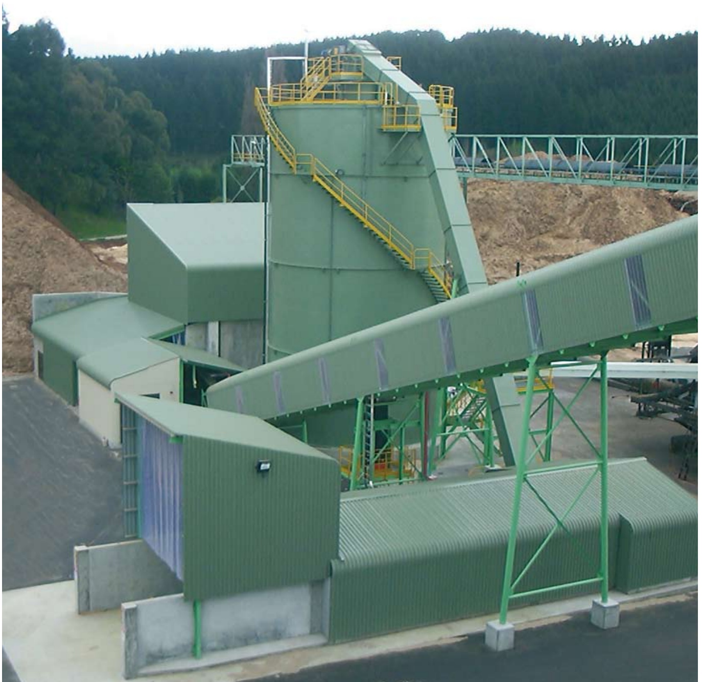
Shavings Reception and Conveyors - 800m 3 Silo - 600m 3 Saxlund Pull Floor
