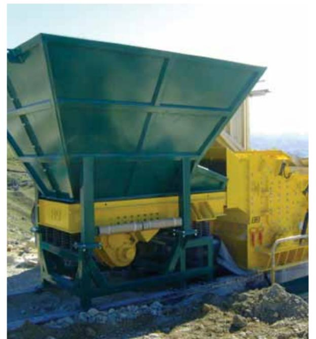
SCS built hopper, feeder and 1010 Impactor during installation at Amuri Lime in North Canterbury.
