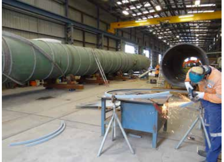
Boiler Stack during fabrication in Nelson
